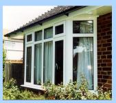
Figure 88: Unequal sightlines are harmful to the appearance of a building as they lack harmony and balance.
