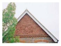
Figure 72: Handmade tile hanging
