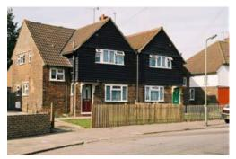
Figure 42: Brook Road Merstham - example of weatherbording, painted a dark colour
