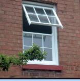
Figure 90: Mock sashes are disruptive to the building form and so should be avoided.
